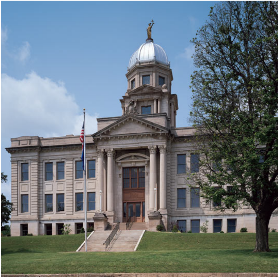
Aluminum-clad wood window with historic profile at the Jackson County Courthouse
