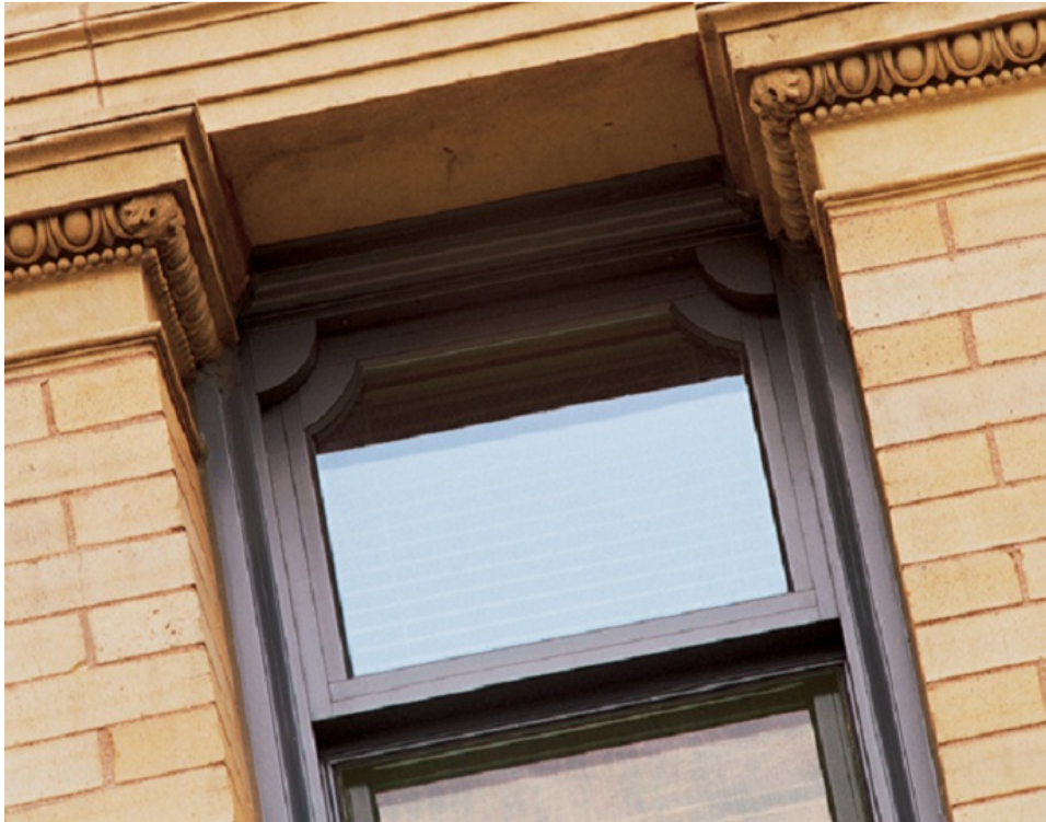
Aluminum-clad wood window with custom profile at the University of Minnesota
