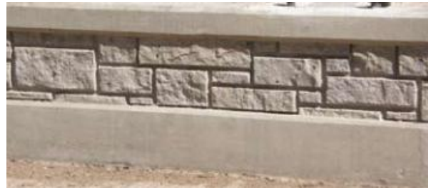
Figure 11. Possible concrete texturing of separation rail.
