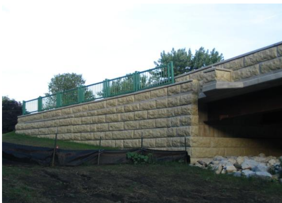
Figure 12. Example of a massive abutment and wing.
