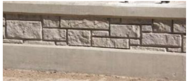
Figure 11. Possible concrete texturing of separation rail.
