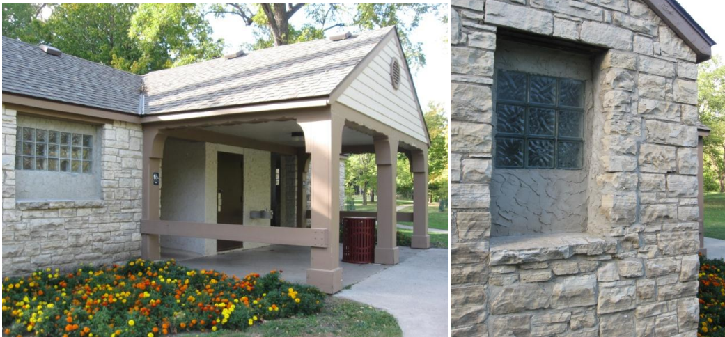
Figure 8. The Brookside Park restroom building inspired the aesthetic treatment for bridge concrete.
