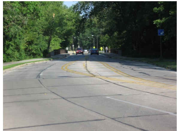
Figure 18. Bridge Approach at East End.
