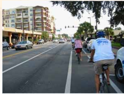
A “road diet” project converted Edgewater Drive in Orlando, FL from a 4-lane undivided roadway to 2-lanes with center turn lane and bicycle lanes.
