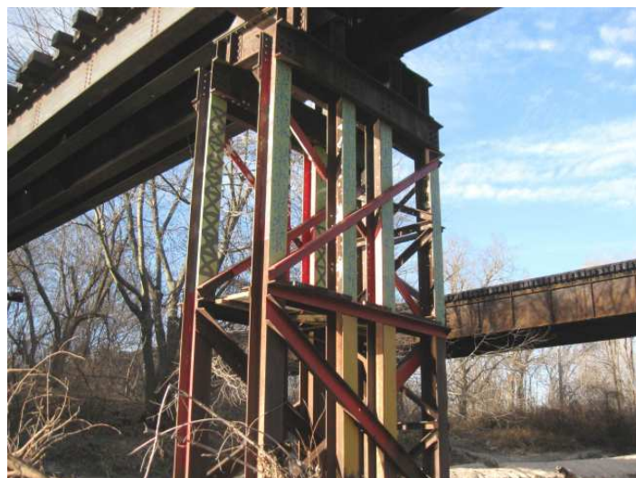
Figure 9. Pier 3 in Stream.
