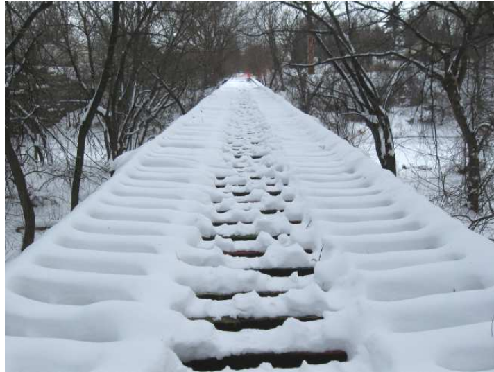
Figure 1. Top of Bridge Deck Looking East.
