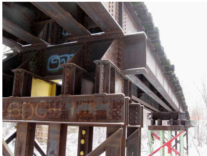
Figure 8. Pier 2 and Profile View, South Side.
