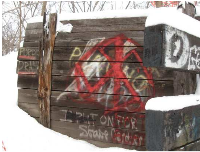
Figure 4. West Abutment Wingwall.
