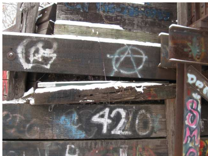
Figure 6. Bad Planks in West Abutment.
